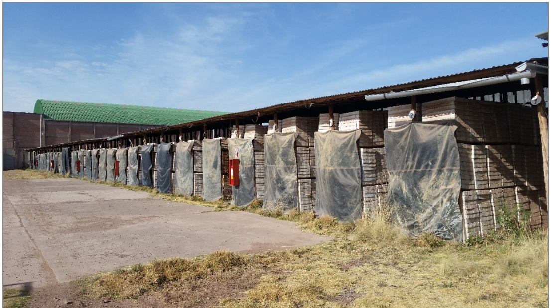
Figure 11-20: Juliaca core storage facility (2) (GRE, 2017)
