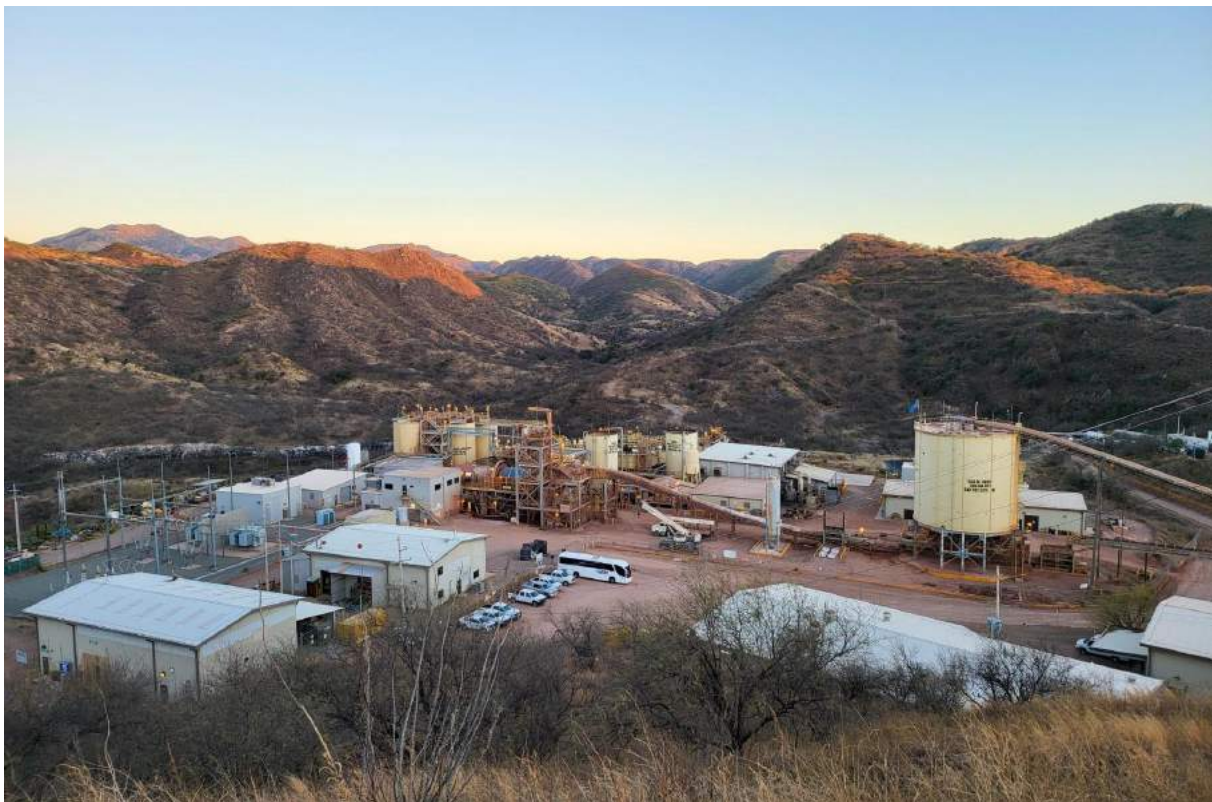
Figure 17-1: Mercedes Mine – Process plant
