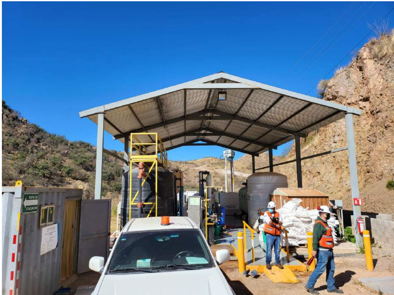
Figure 18-7: Water treatment plant
