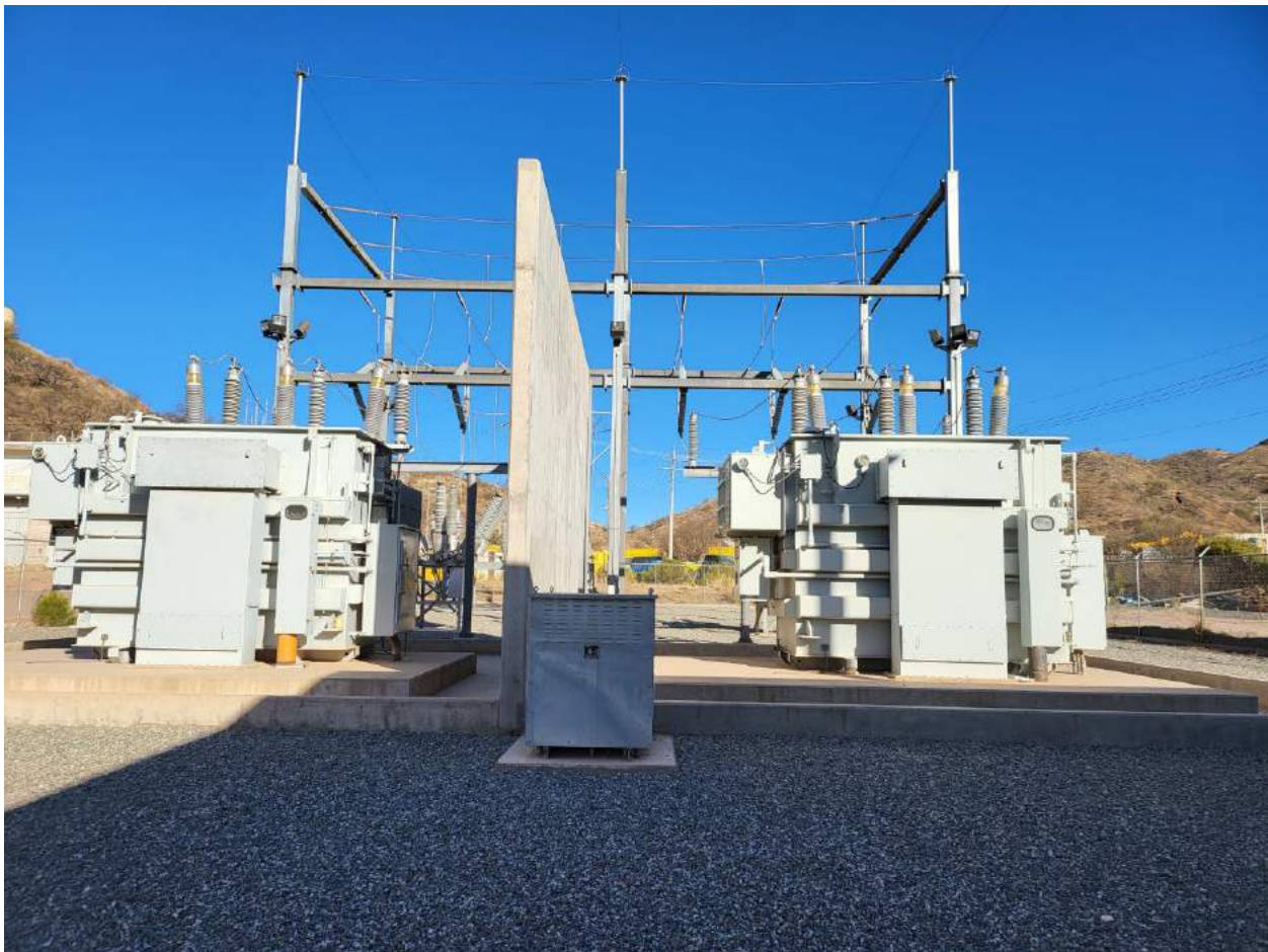
Figure 18-4: Power supply - Step down to 13.2 kVA
